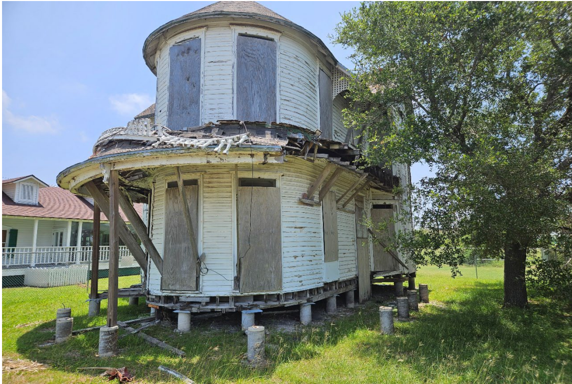
Northeast corner. Damage to Balusters and porch cover.
