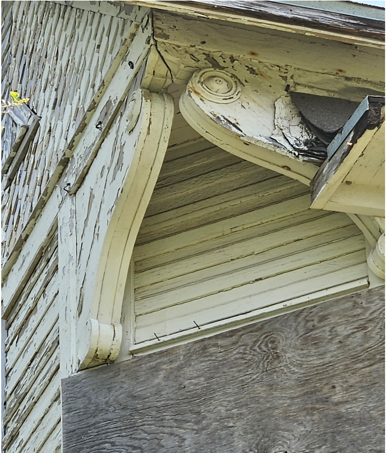
Corbel and roof edge dry rot.
