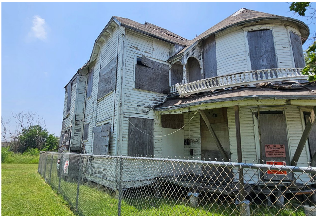
Southeast corner. Siding damage.
